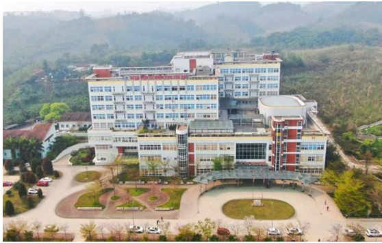
Figure 1.2: Consolidated model – Lao Cai No. 1 General Hospital (Source: Lao Cai No. 1 General Hospital)
