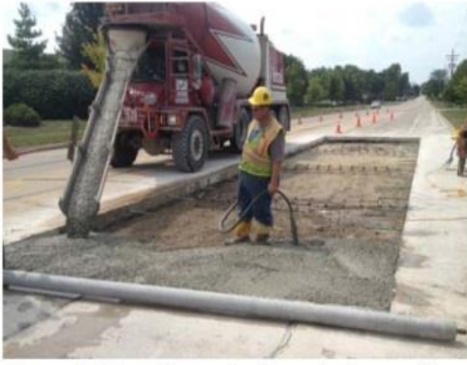
Figure 1.2. Internal maintenance CONCRETE CEMENT road surface
