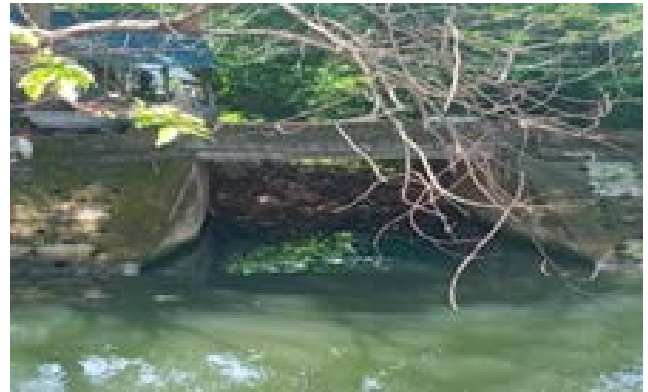
Fig. 5. Outlets of combined sewers into An Cuu River at Ton Quang Phiet Str.
