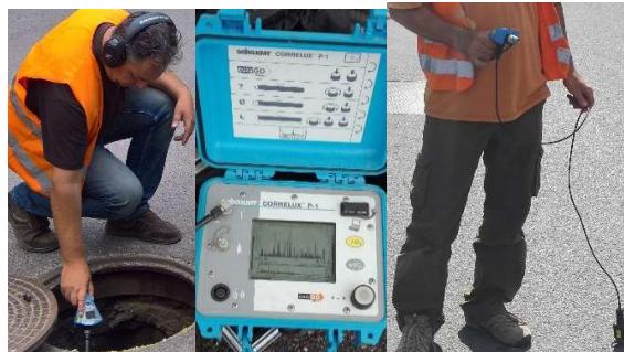
Figure 8. Leak locator (left and right) and Digital correlator for leak location on pipe (middle).
