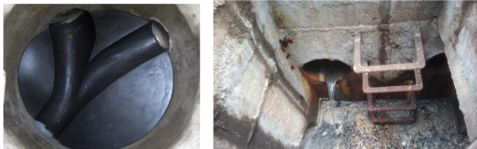
Figure 4: Image of Manhole with Invert in left and manhole without Invert in right
