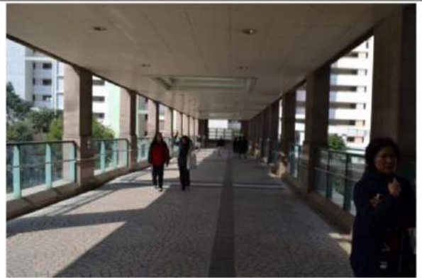
Picture D-4: Inside of the walkway bridge on Po Fung Rd.
