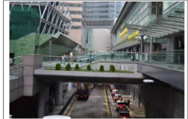
Picture A-5: Walkway bridge connecting to IFC Mall
