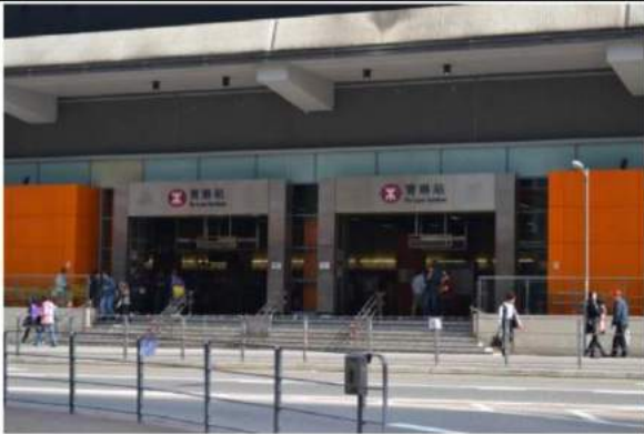
Picture D-1: Po Lam MTR Station
