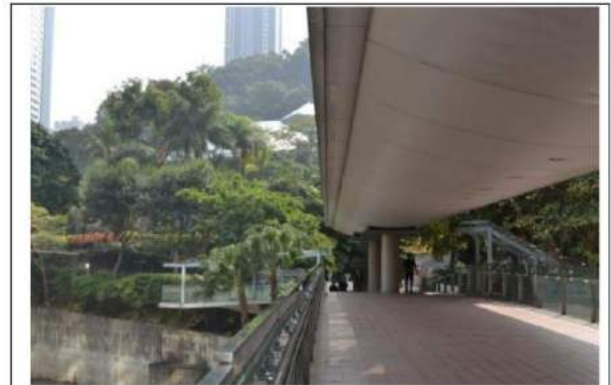
Picture A-6: Walkway bridge connecting to Hong Kong Park
