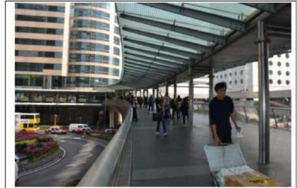
Picture A-4: Walkway bridge above Connaught Rd.
