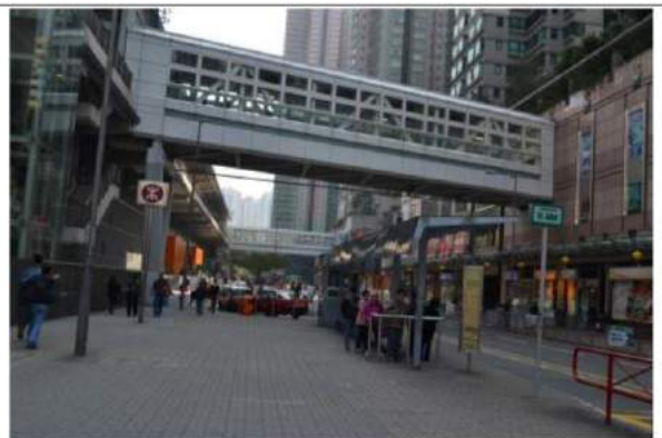
Picture D-5: Walkway bridge connecting from MTR to Metro City 1
